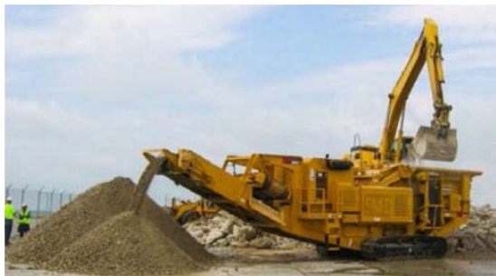
Crushing machine being loaded with construction debris by an excavator.
