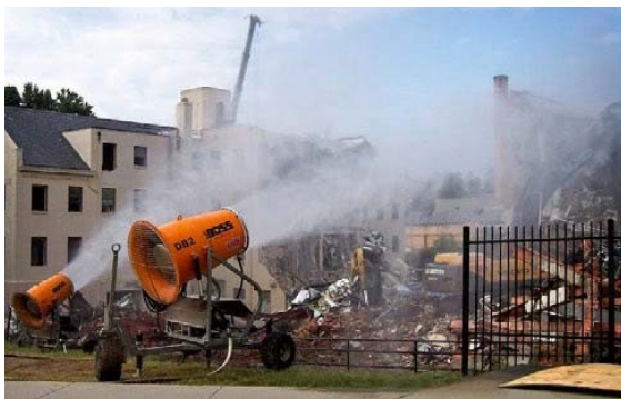
Atomized misting cannons, like the DustBoss unit pictured, are an effective way to suppress silica dust.
