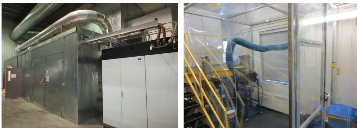
Figure A4. Work area containment
